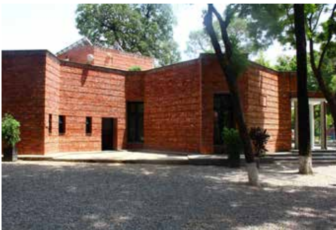
Brickwork of new CDH
