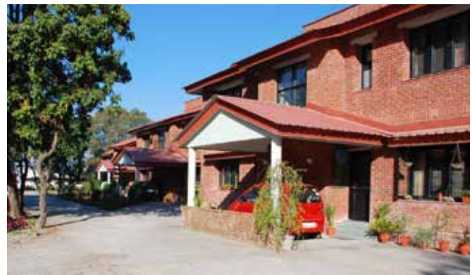
Hathikhana Houses southern elevation - Roopak Kothari 2008
