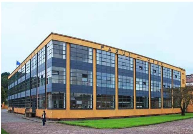
The Fagus-Werk Factory in Alfeld, Germany, was designed by Gropius and Adolf Meyer in 1911 and is considered one of the earliest examples of modern architecture. The ten-building complex is noted for its glass-and-steel curtain walls and support-free corner windows and was named a UNESCO World Heritage Site in 2011
