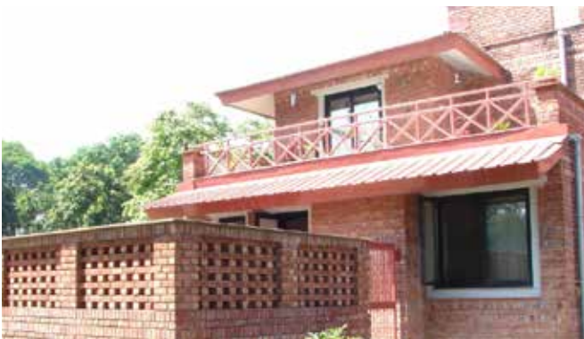
Main Field House south side. Overlooks the field till the aqueduct.
